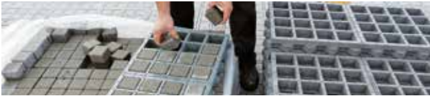
Insertion of the paving stones in the TTE® element
