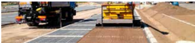
Insertion of the filling with a paver
