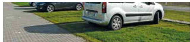
Green company parking area after 10 years of daily use
